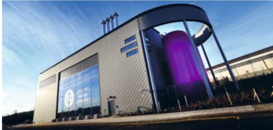
The Gateshead Energy Centre, on the town's Quarryfield Road
